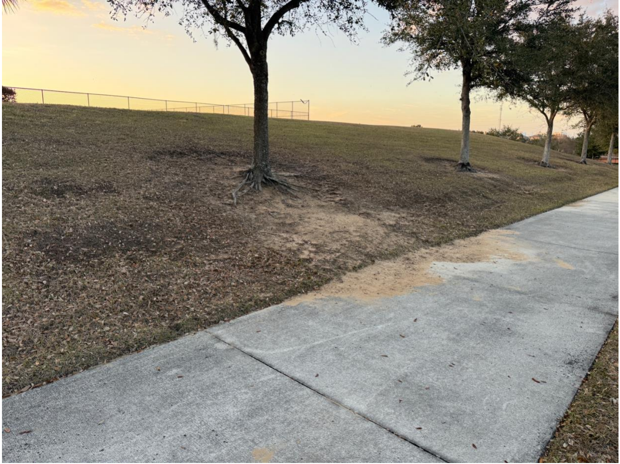
Washout / Erosion of dirt on trees behind the pool
